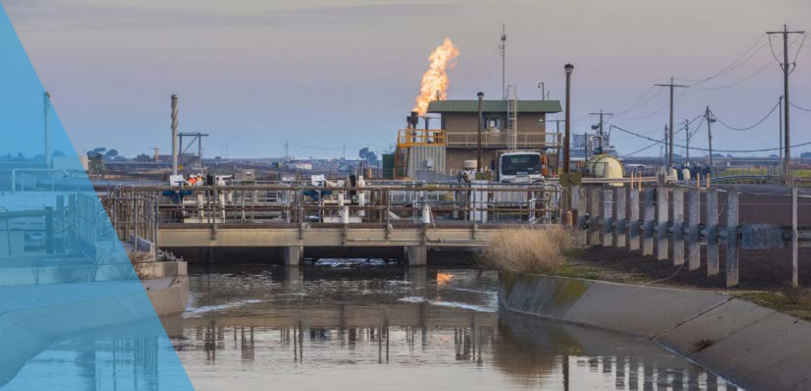
Water treatment plant (photo courtesy of Melbourne Water)
